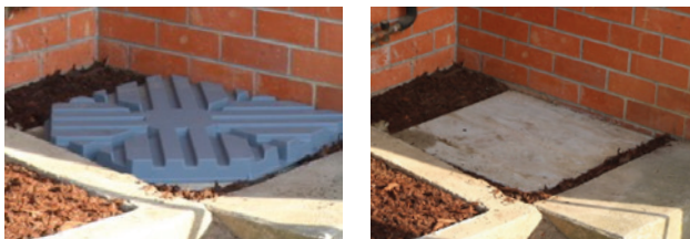
Figure 1: Concrete or heavy duty plastic slabs to be placed under the storage tank and/or heat pump.
